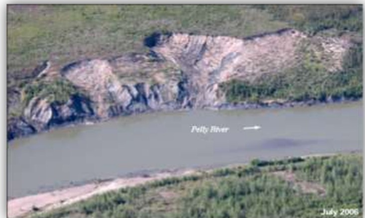
Figure 9. Oblique aerial photograph of a retrogressive thaw slump (#5 in Fig. 3) that was contributing sediment to the Pelly River in 2006. This landslide has been active and increasing in size since at least 1989. View is to the south. Estimated width of main failure is approximately 200 m.
